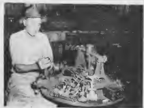
Small valves need reclaiming just as much as big ones. Augustinus Figarua (above) is seen repairing small screw valves.
